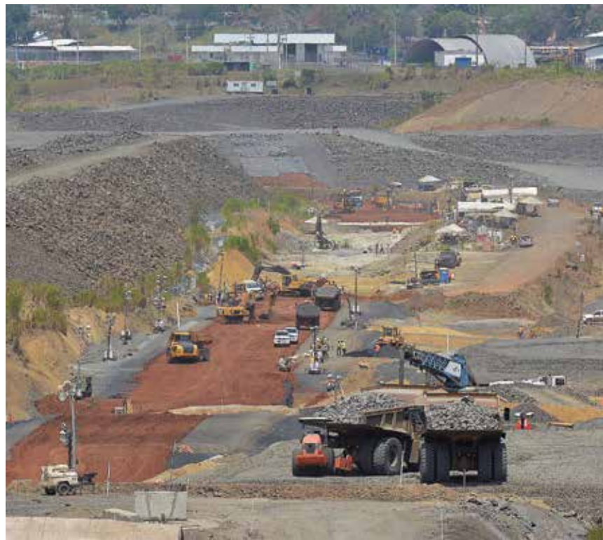
Ongoing work to place the impervious clay core for the Borinquen 1E dam.
