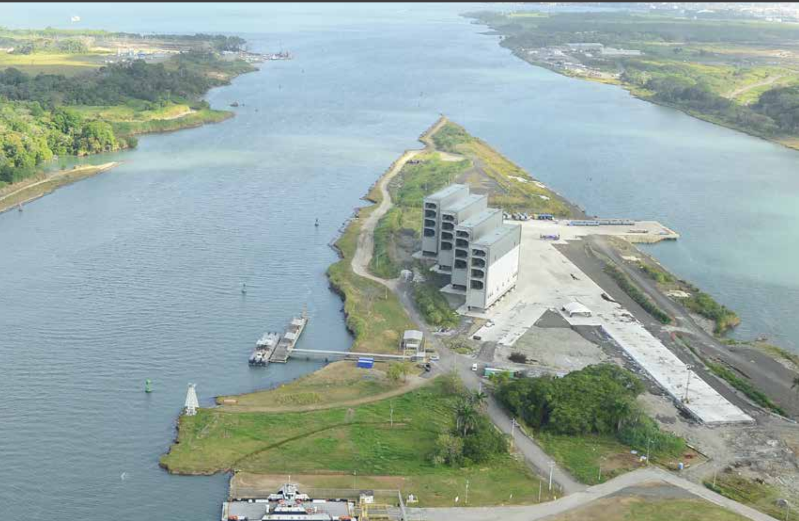
The first four rolling gates will be installed in the Atlantic locks middle chamber.
