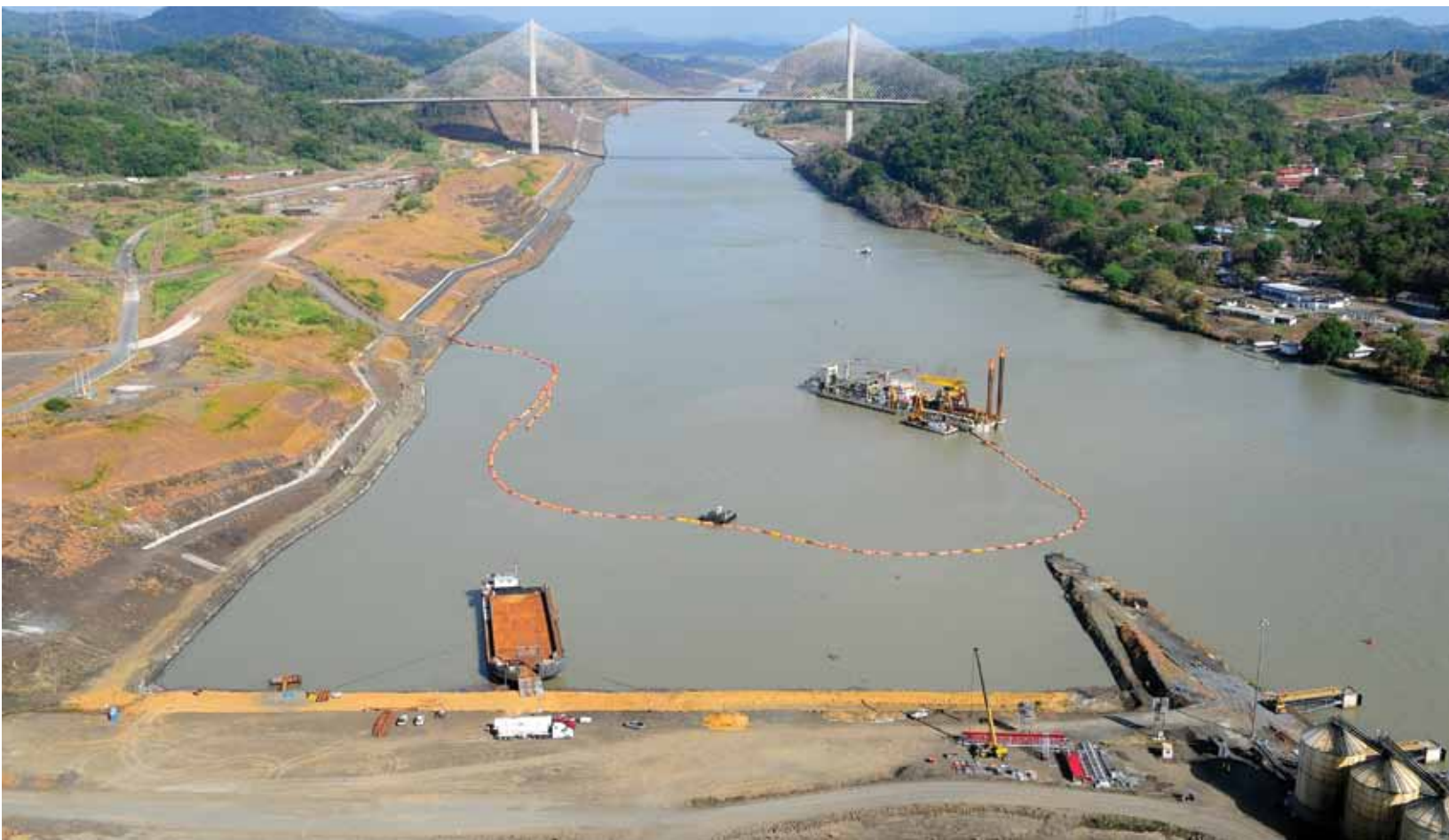
Dredging of the north entrance to the Pacific Access Channel.
