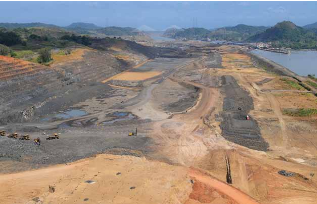
Construction work for the foundation of the Borinquen dams.
