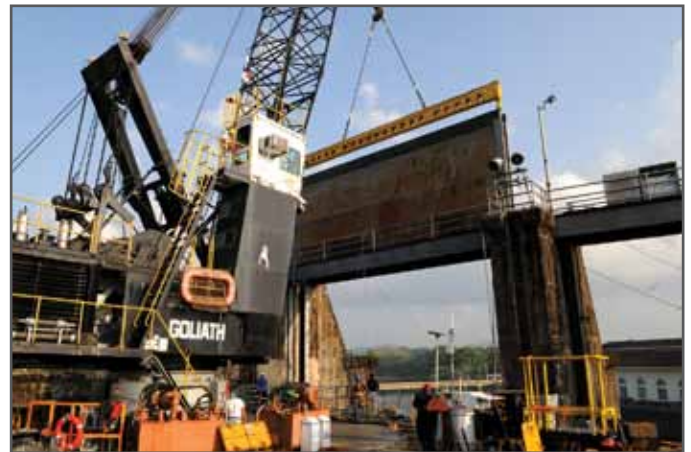
Modification of Gatun spillway gates
