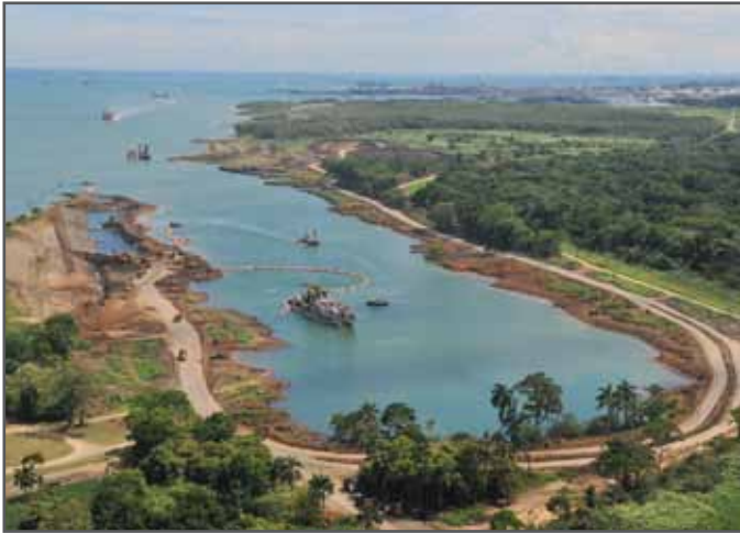
Dredging work on the Atlantic side
