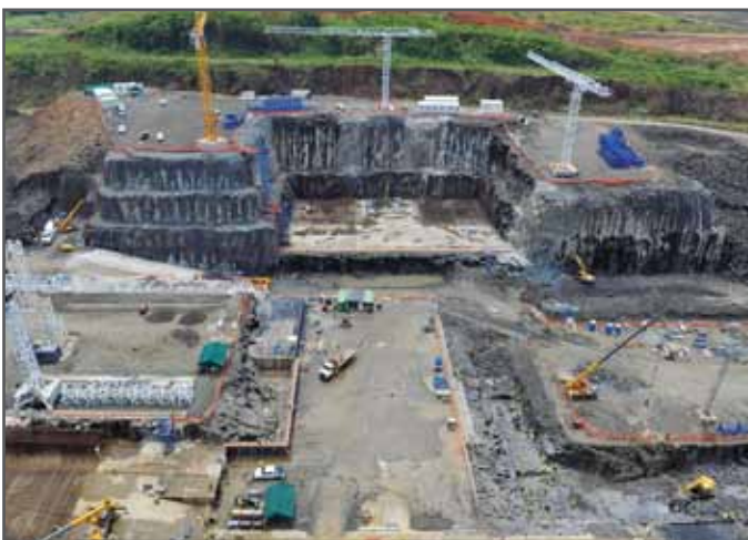
Work in the area of one of the Third Set of Locks gate recesses on the Atlantic side
