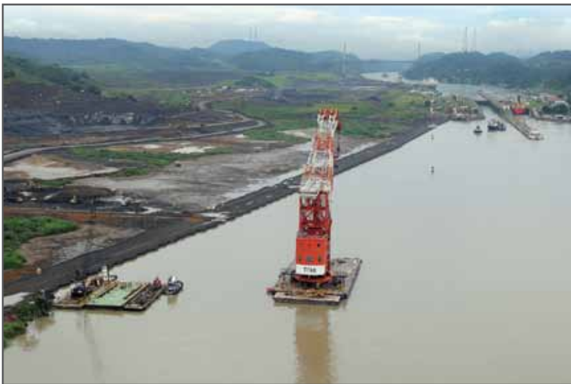
Borinquen Dam cofferdam
