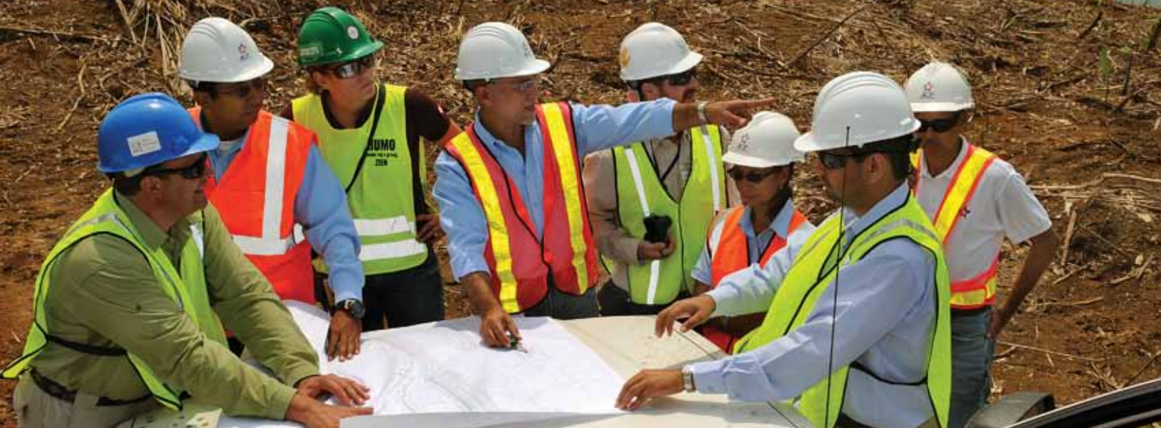
The Atlantic dredging team and contractor personnel check project drawings on the field.
