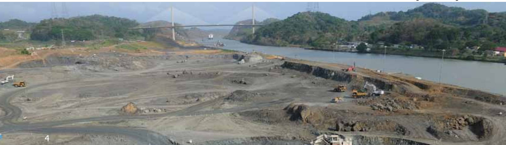
PAC-3 work area with Centennial Bridge in the background.
