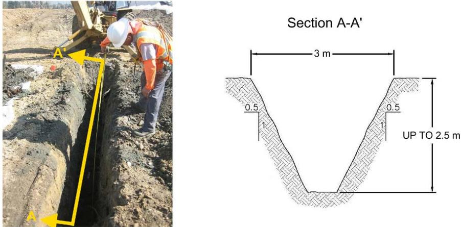
Fig. 2. Typical investigation trench cross section.
