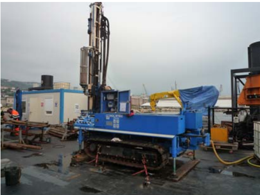
Figure 2: Adapted on-shore track-mounted geotechnical drilling rig working from jack-up deck
