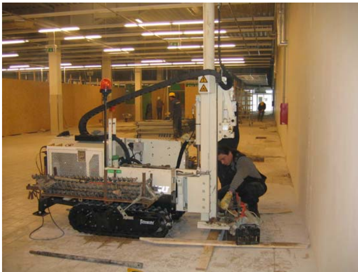
Figure 3. Anchored Geoprobe® soil probing machine with CPT.
