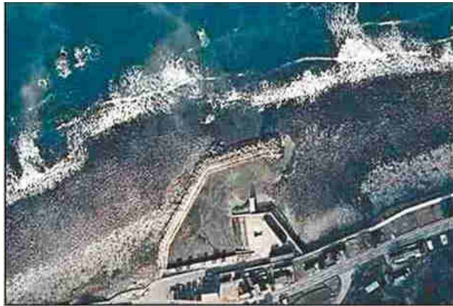
Tsunami observation meter inactive due to seafloor exposure
