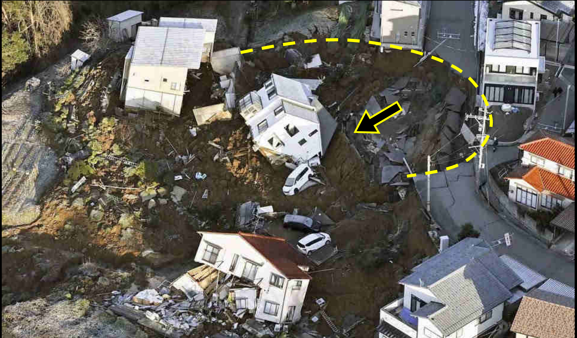
collapsed houses, cars, roads in Kanazawa Source: Kvodo/via REUTERS
