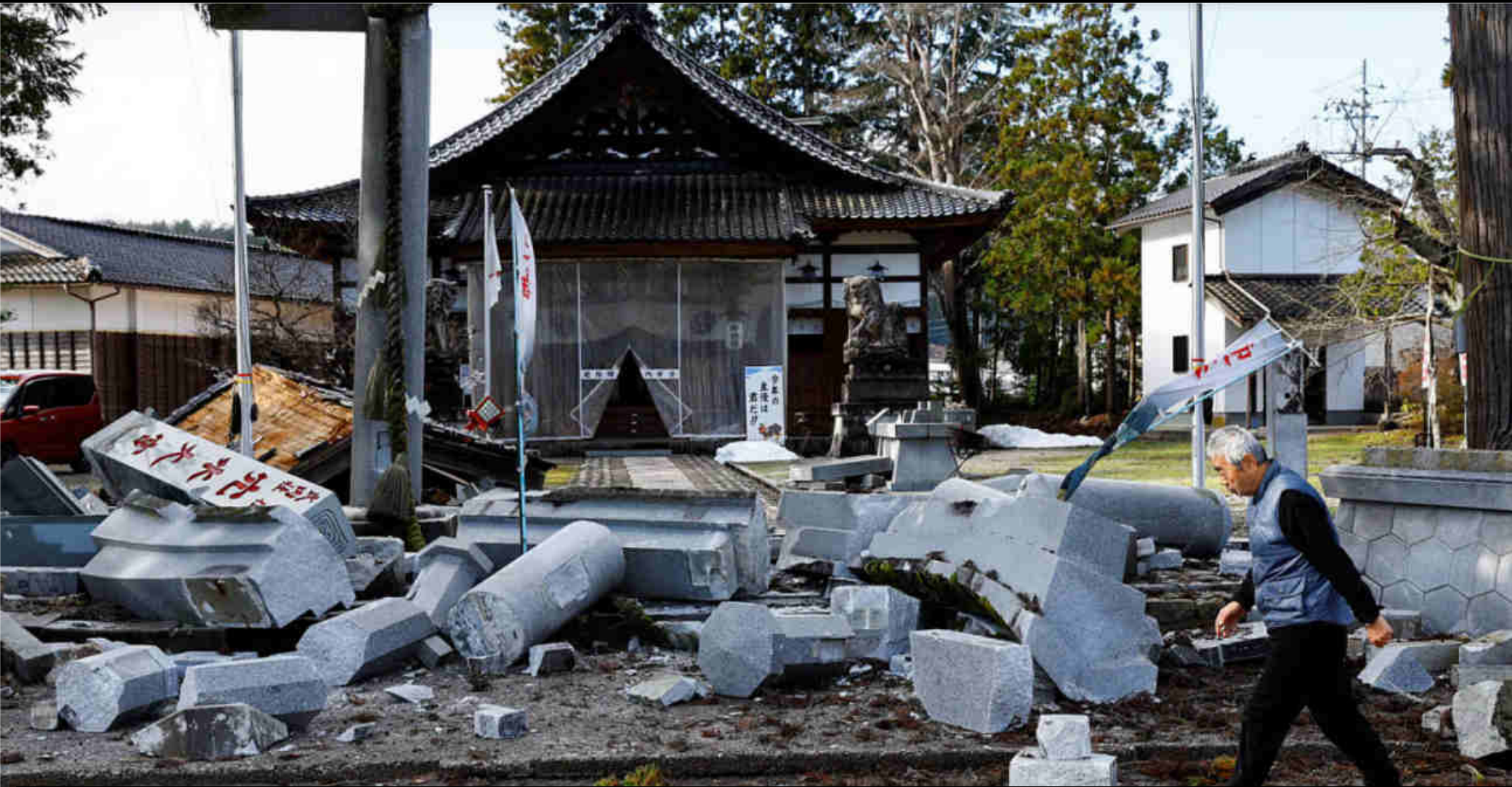
A damaged shrine in Ujima
