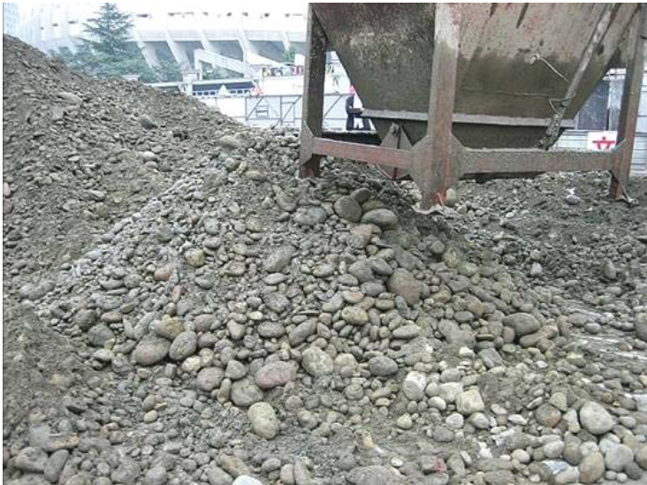
Fig.1 Cobbles exposed during pit excavation
