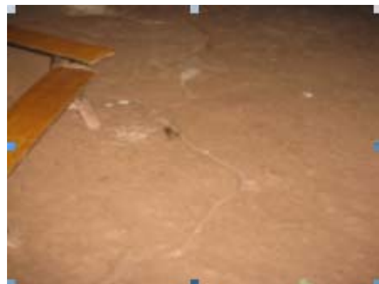
Fig.6 Cracks in the residential area
