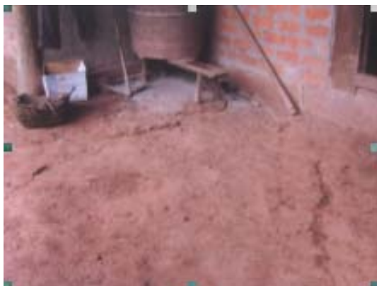
Fig.6 Cracks in the residential area
