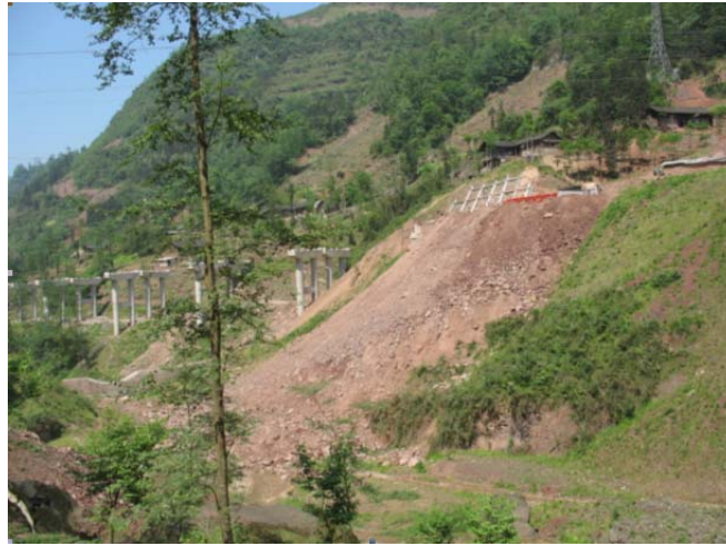
Fig.7 a electricity transmit in the top of the ancient landslide
