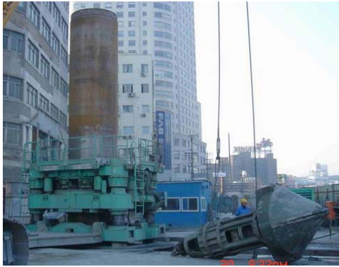
Fig.6 360° rotation drilling and cutting machine
