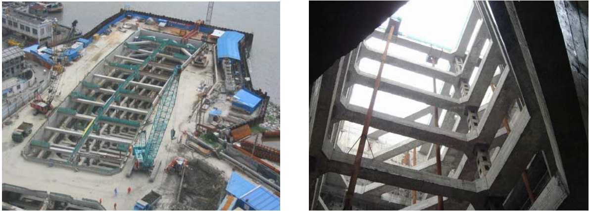
Fig.12 Deep excavation and strut system
