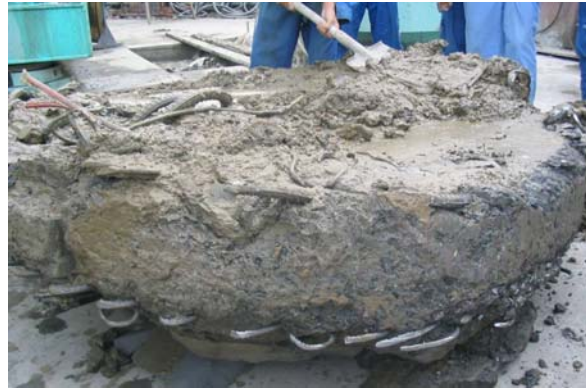
Fig.7 Removal tunnel segment
