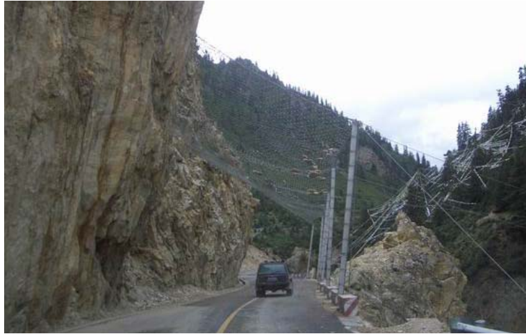
Fig.1 A rock slope on a mountain road in the west regions of China.
