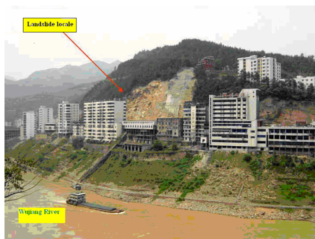
Fig.1 Panoramic view of Wulong ‘1 May’ landslide area
