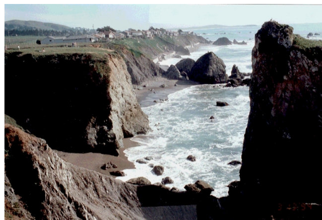
Figure 2: Franciscan melange at Coleman Beach, California. Blocks form erosion-resistant headlands and buttress up-slope weaker block-poor melange. Several homes are threatened by cliff-top retreat of block-poor melange.
