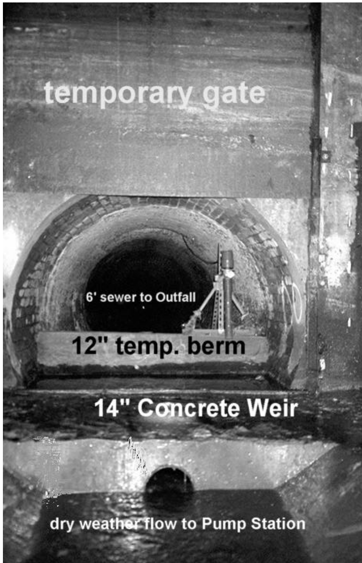
Figure 7 – Overflow Structure, Looking Downstream.
