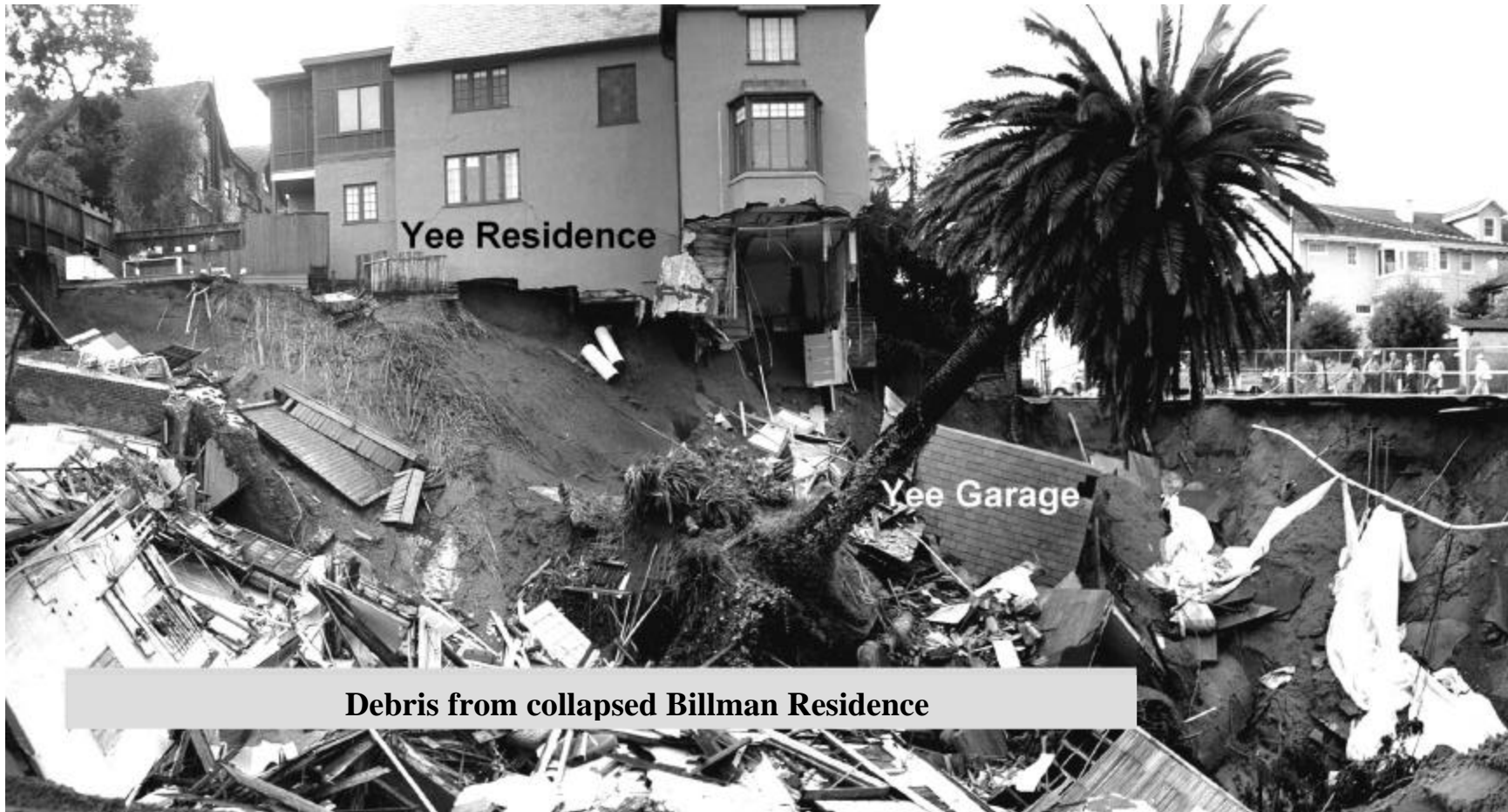
Figure 2 – Aftermath of the Sea Cliff Incident: a 200 foot diameter and 40 foot deep pit containing the debris from the collapsed Billman residence. Yee residence in background.
