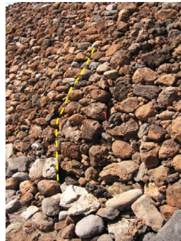
Figure 18. Post-earthquake photo near NE corner of Pu'ukoholā shows bulging of face of wall (indicated by yellow line).
