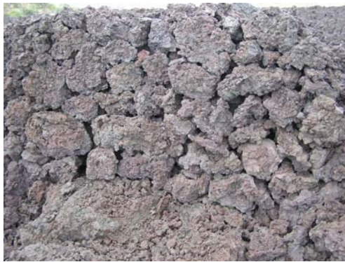
Figure 3. Rock wall of loosely placed a'a clinker blocks.
