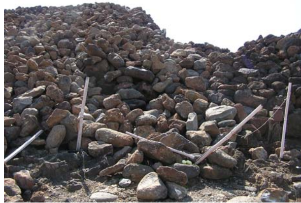
Figure 16. Post-earthquake view of collapsed entrance.
