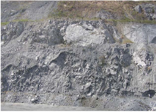
Figure 8. Rock exposed in slope excavated within San Andreas fault zone, Northern California. Sheared rock surrounds hard blocks of relatively intact rock. Blocks range between centimeters to tens of meters in size. (Photo: E. Medley/Geosyntec Consultants).
