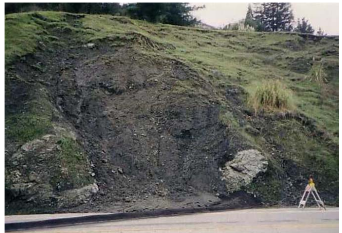
Figure 4. Blocks in Franciscan melange buttress slope between landslides in sheared shale. (E. Medley/Exponent)
