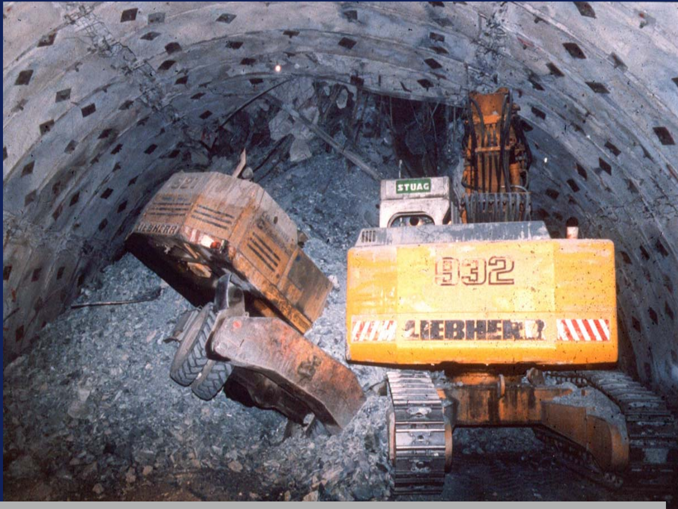
Galgenberg Tunnel, Austria
