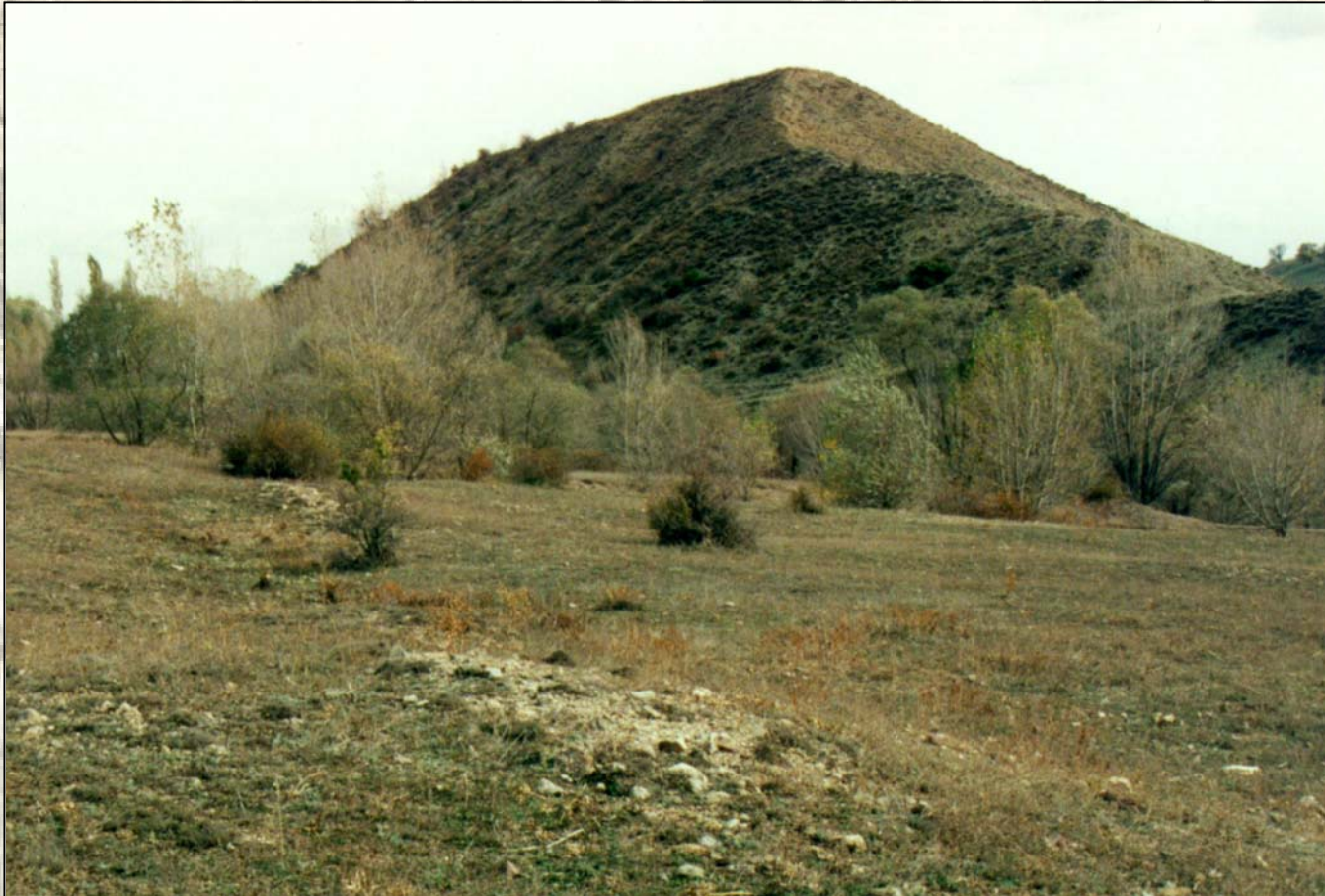
North Anatolian Fault Zone, Turkey Fault Escarpment of Active Segment, near Bolu Tunnel
