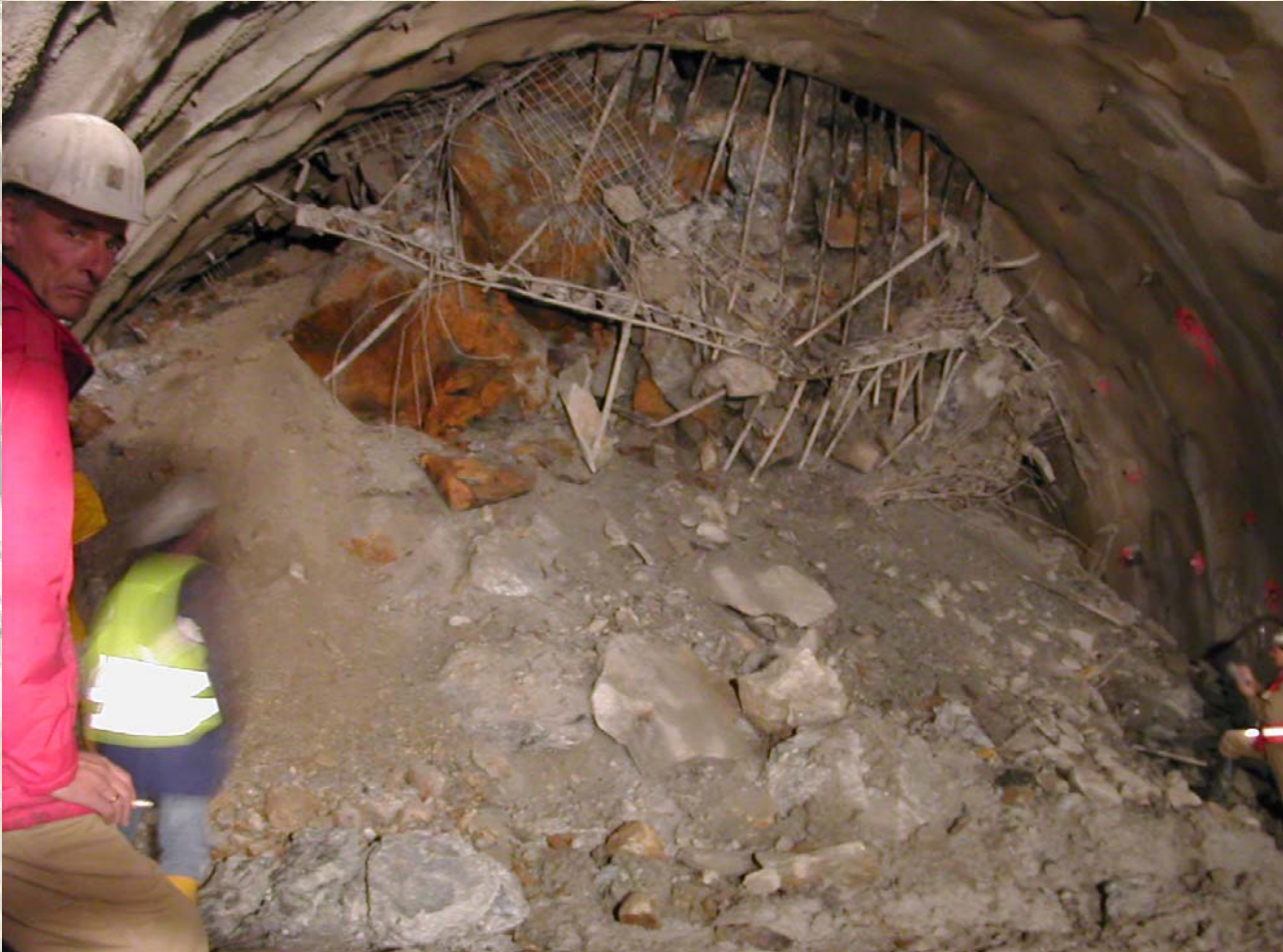
Herzogberg Tunnel, Austria
