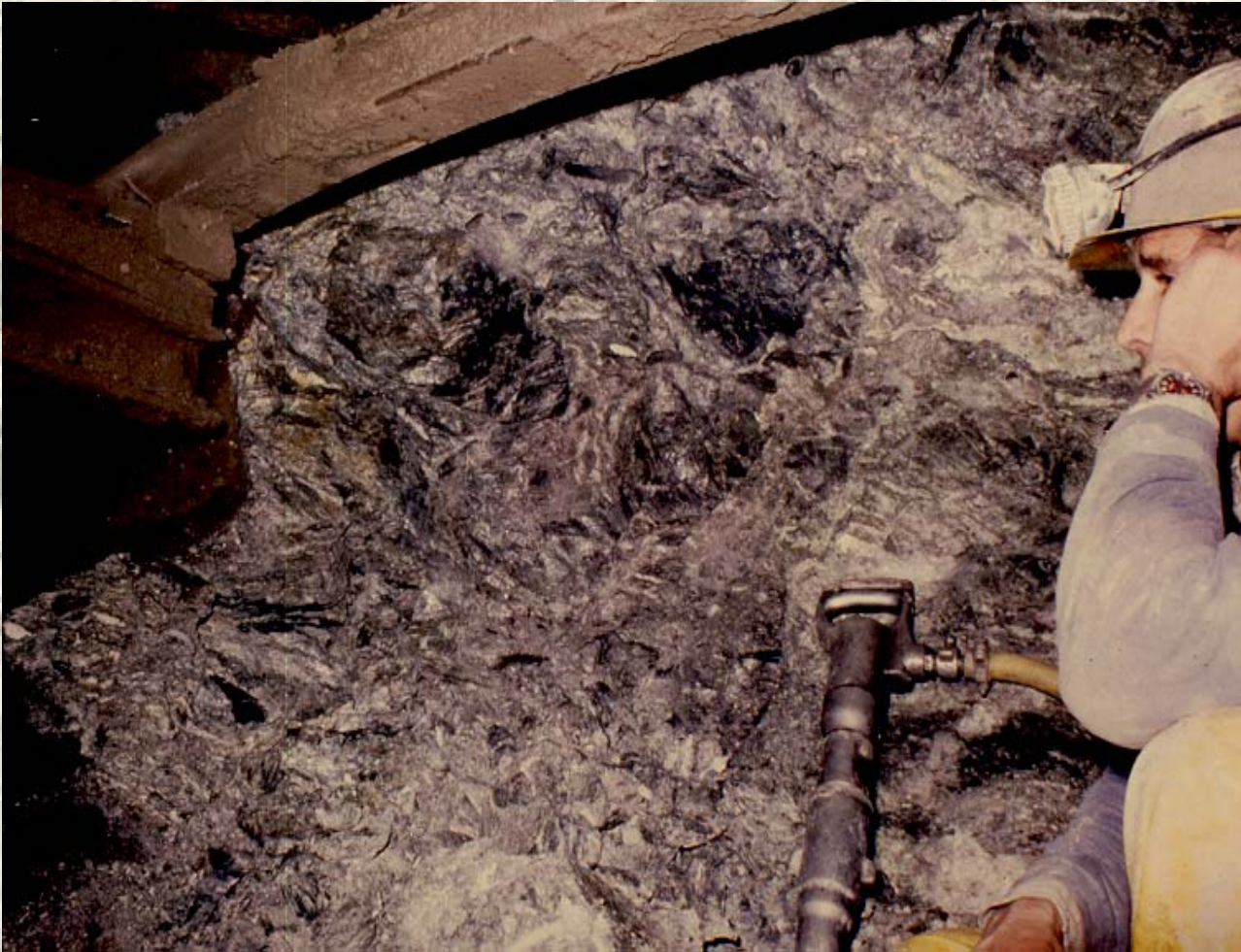
Herzogberg Tunnel, Austria
