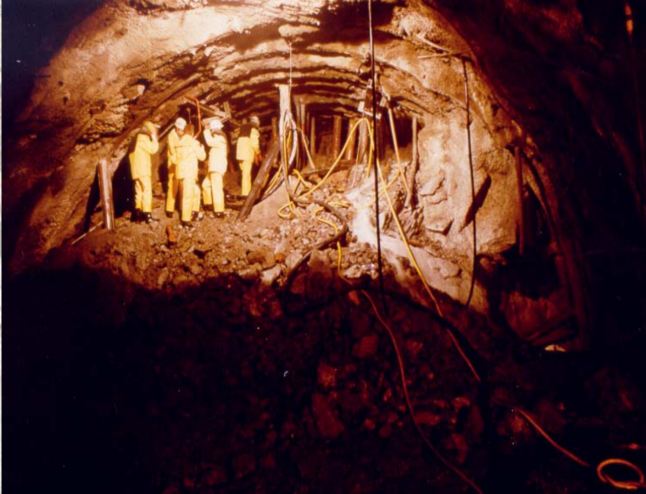
Herzogberg Tunnel, Austria
