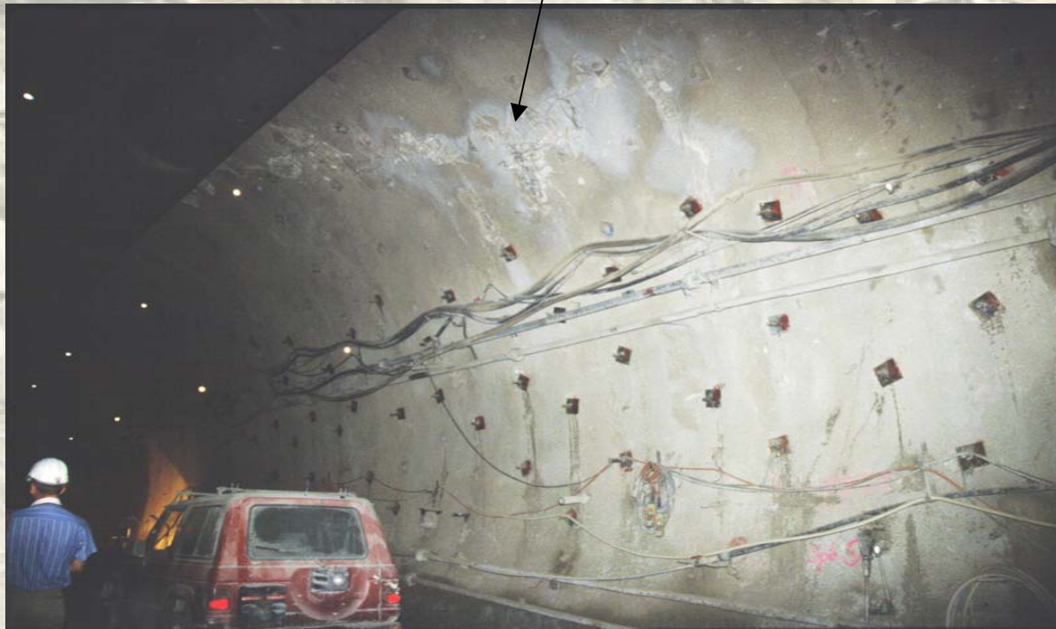
Tunnel Spital, Austria
