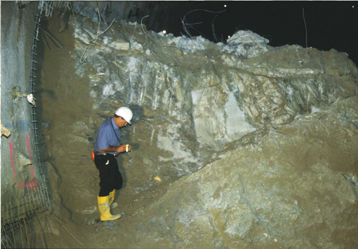
Tunnel Spital, Austria
