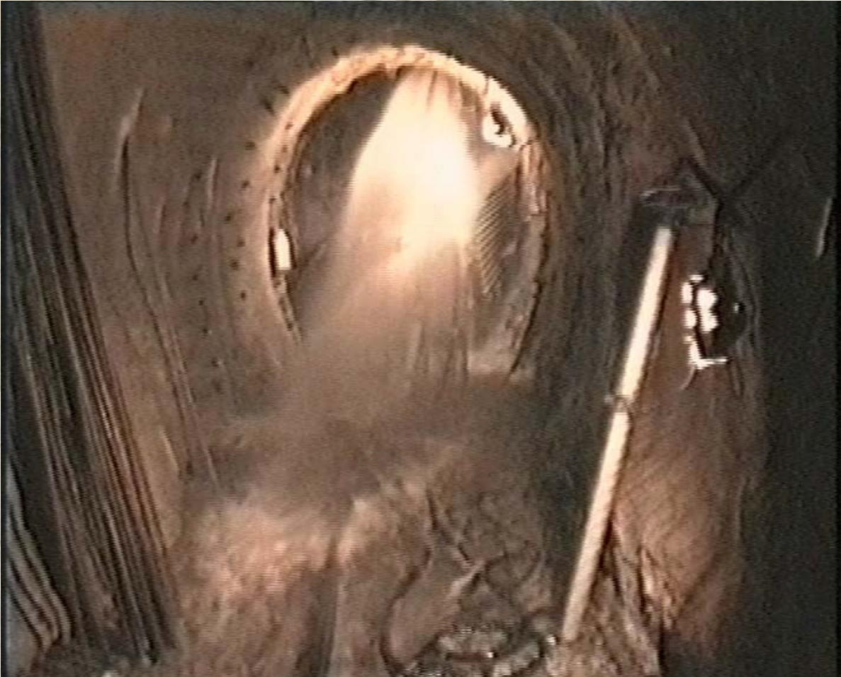
BASO CHHU TUNNEL (Bhutan, 1999, 450 l/s)
