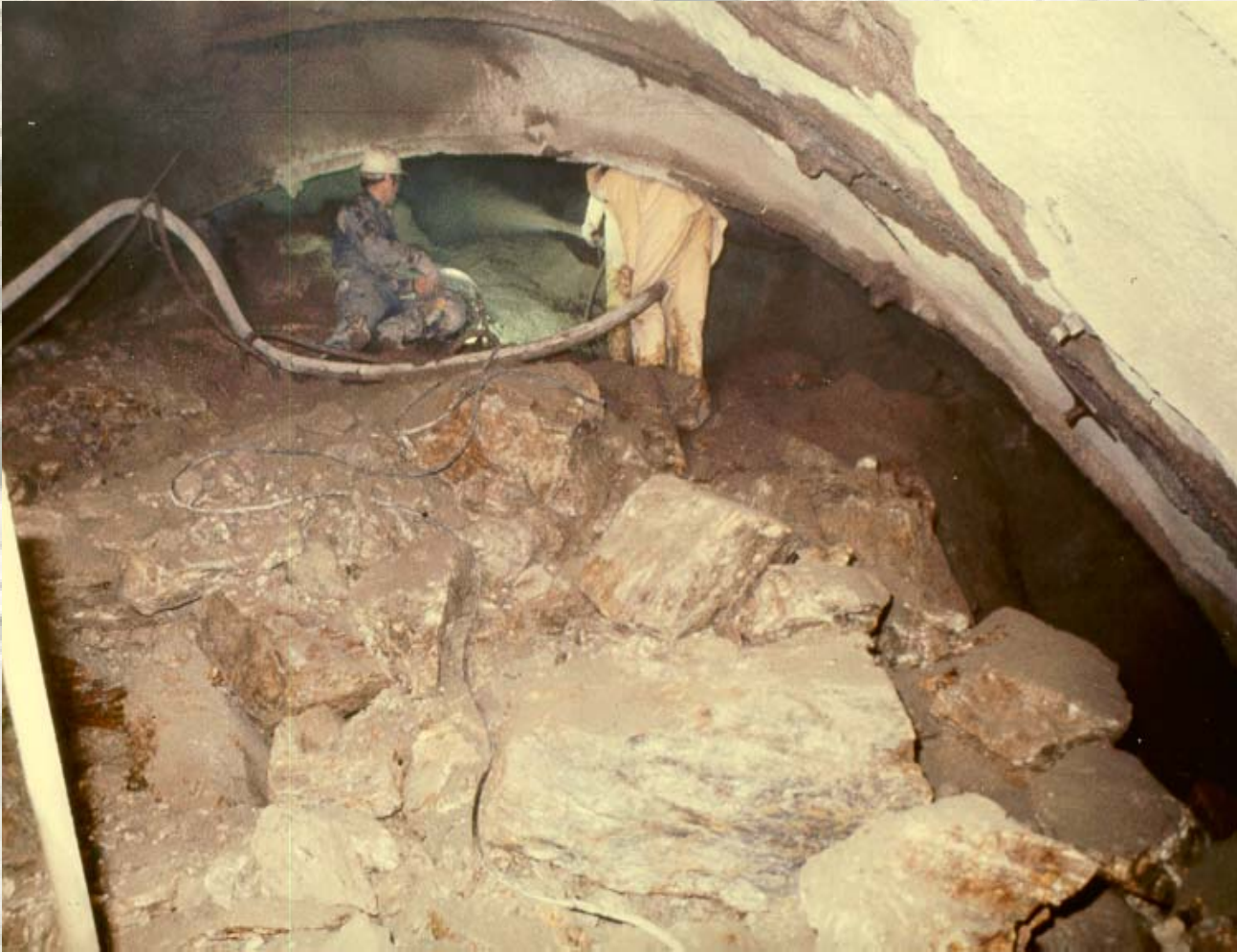
Herzogberg Tunnel, Austria
