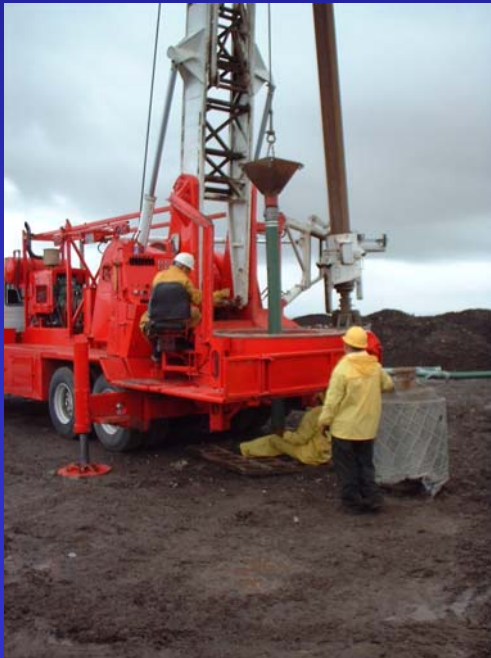
3. Place tremie pipe in borehole
