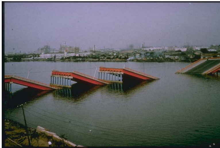
Figure 1.7: Failure of Showa Bridge after NISEE.
