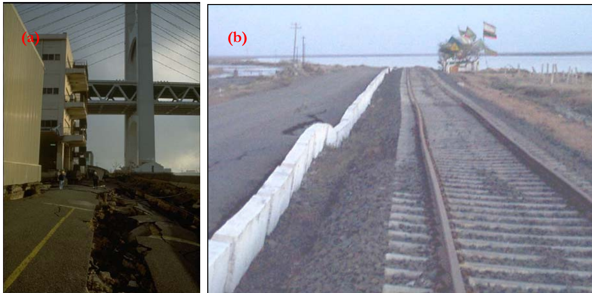
Figure 1.5 (a): Surface observations of lateral spreading at a bridge site in 1995 Kobe earthquake after NISEE; (b): Navalakhi port in 2001 Bhuj earthquake, Madabhushi et al (2001).
