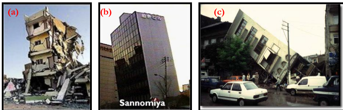
Figure 1.1: (a) Failure of a residential building during the 2001 Bhuj earthquake (India); (b): A highrise building during the 1995 Kobe earthquake, after U.C. Berkeley (1995); (c): Tilting of a building during the 1999 Koceli earthquake (Turkey), after EERI (1999).
