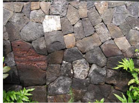
Figure 4. Rock wall of intricately interlocked massive basalt blocks (Moku'aikaua Church, Kailua-Kona, Hawaii).
