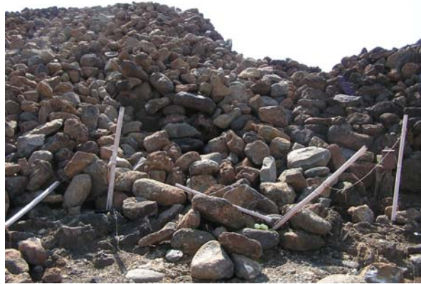
Figure 16. Post-earthquake view of collapsed entrance.
