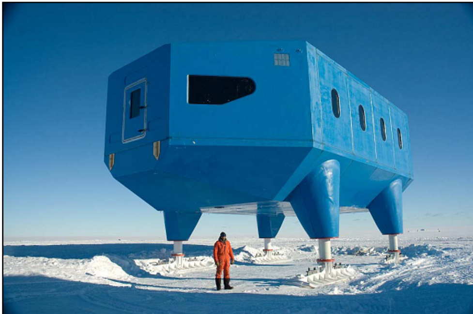
Figure 4. Halley VI Base module (courtesy British Antarctic Survey)
